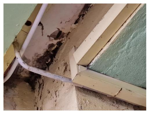
Photo 7: Ingress of water from the roof slab above and presence of mold.
