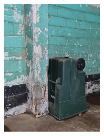
Photo 10: Damage to base of columns with rebar exposure.
