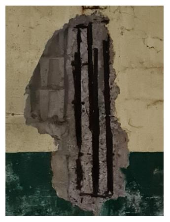
Photo 13: Damage to stiffener column within blockwall.
