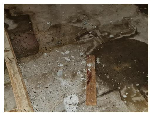
Photo 17, Small chunks of spalled concrete on floor from ceiling above.
