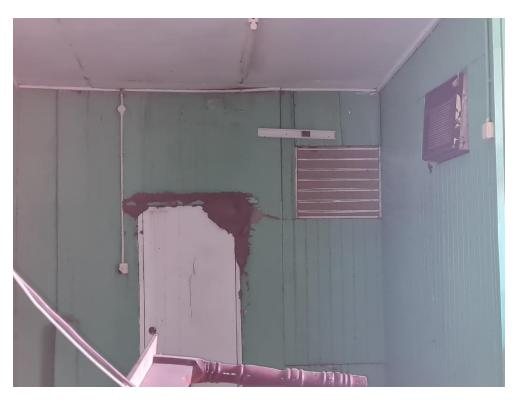
Photo 18. Active termite nest above door in 2 storey office section.
