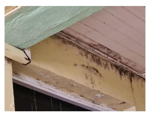
Photo 6: Ingress of water from the roof slab above and presence of mold.
