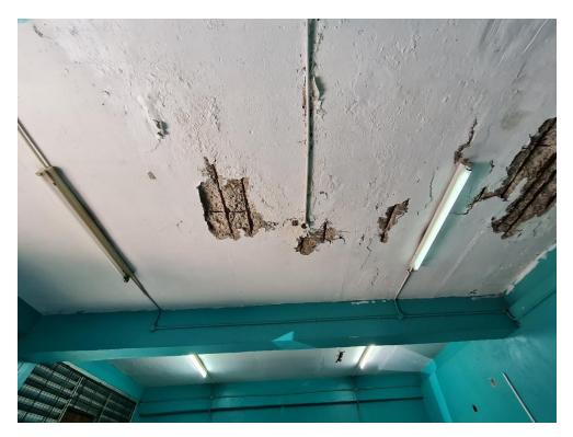
Photo 8: Spalling of concrete from soffit of concrete roof slab.
