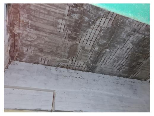
Photo 16: Damaged and actively spalling concrete slab soffit with exposed rebar.
