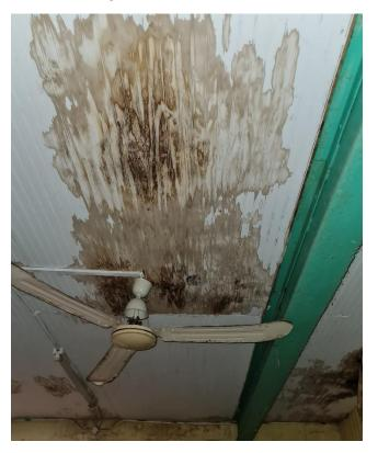
Photo 14: Water and mold damage to timber plywood ceiling. Note proximity of electrical fan.
