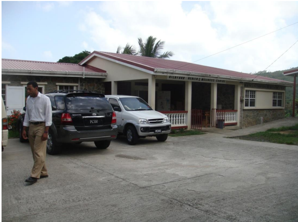
Photo 2.3. Richfond Health Centre, occupied by Dennery Hospital operations
