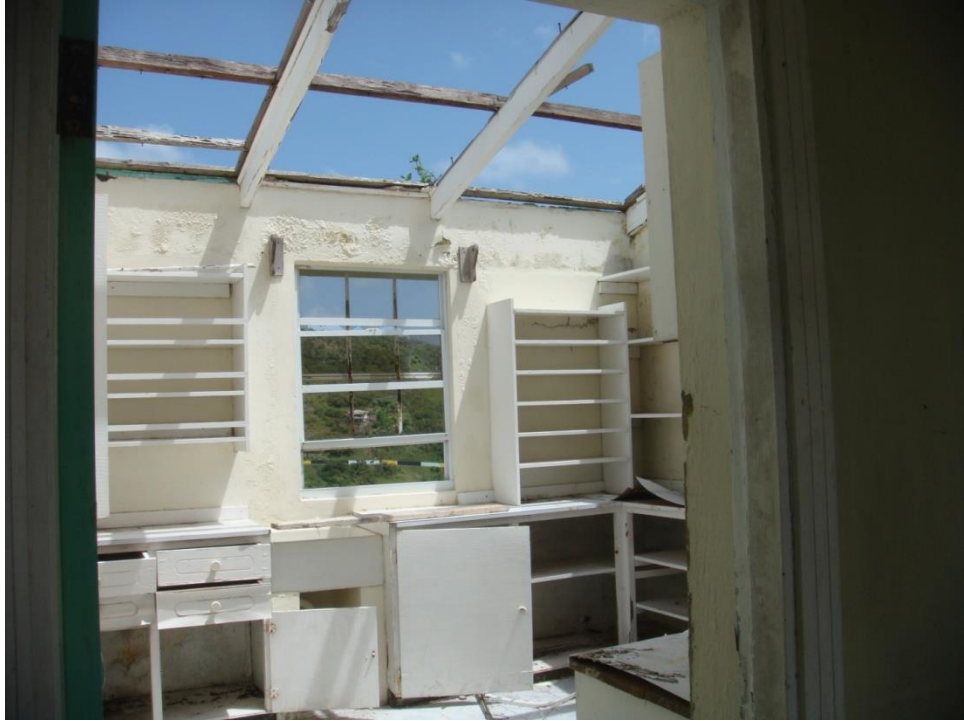
Photo 2.2. View of inside of old Dennery Hospital to be renovated
