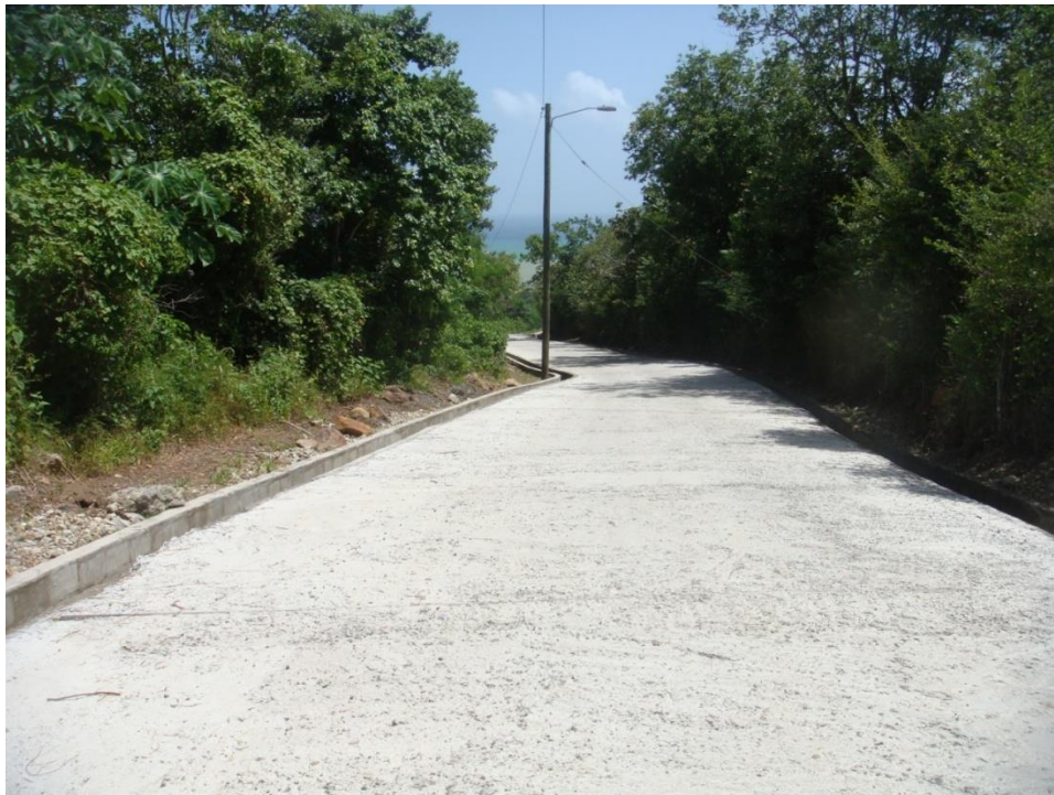
Photo 2.6 . Existing concrete access road past SDA church in Bois Jolie
