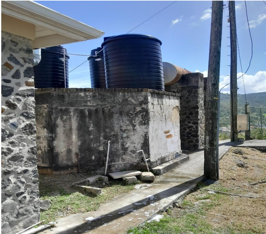
Existing water tank
