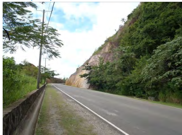
Figure 5.5: The Millennium Highway rock slope failure in zone LL (south) rockfall related to discontinuities
