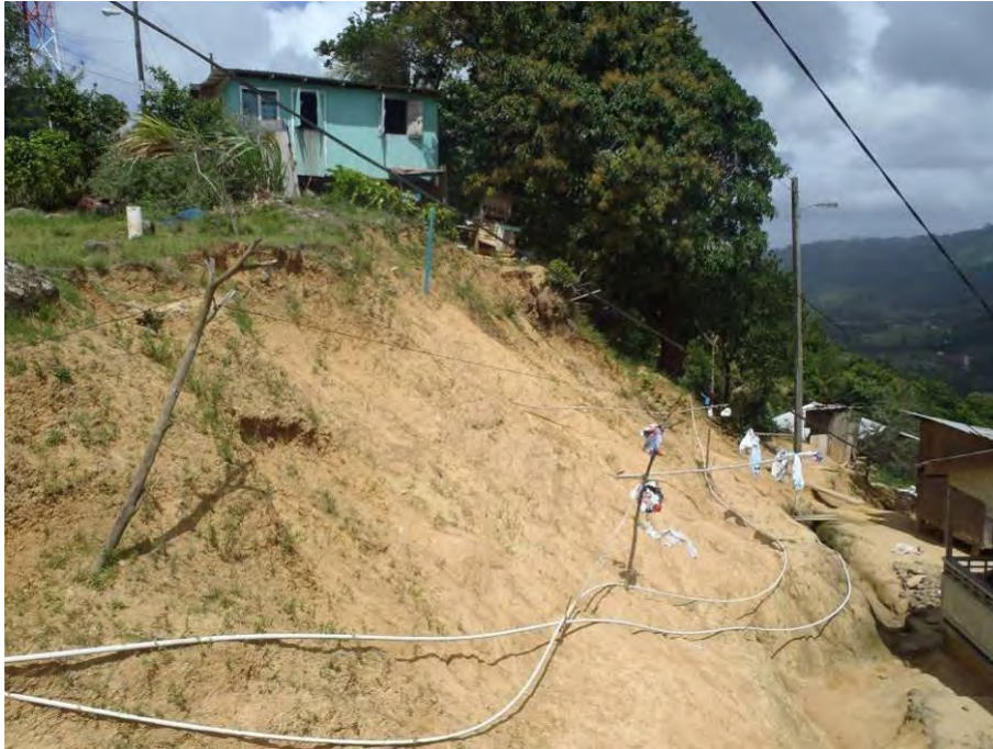
Figure 2.2: Installation completed for 1998 WEMP project recently exposed by a landslide
