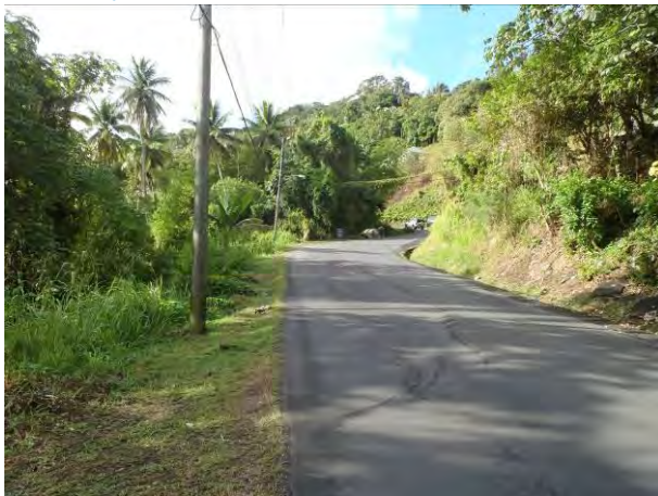
Figure 1.3: Arcuate crack and depression in road caused by landslide at Ti Colon (Ch 22955 – 23000 SB)
