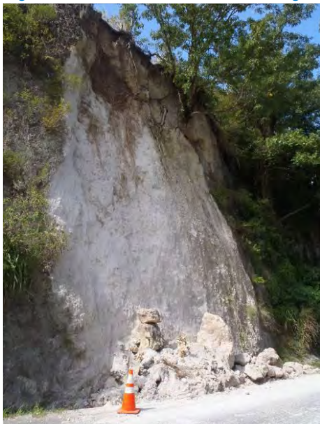
Figure 1.2: Small rock fall onto the highway in zone 7
