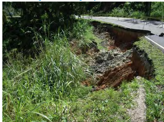
Figure 5.7: translational slide on top of the Barre de L'Isle showing loss of carriageway
