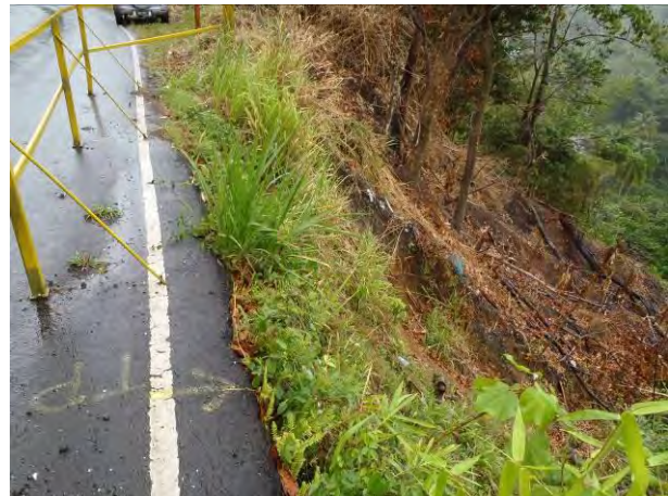
Figure 1.4: Shallow slope failure along road at Site 9 on the Barre de L'isle (Ch 125295 – 125340 WB)
